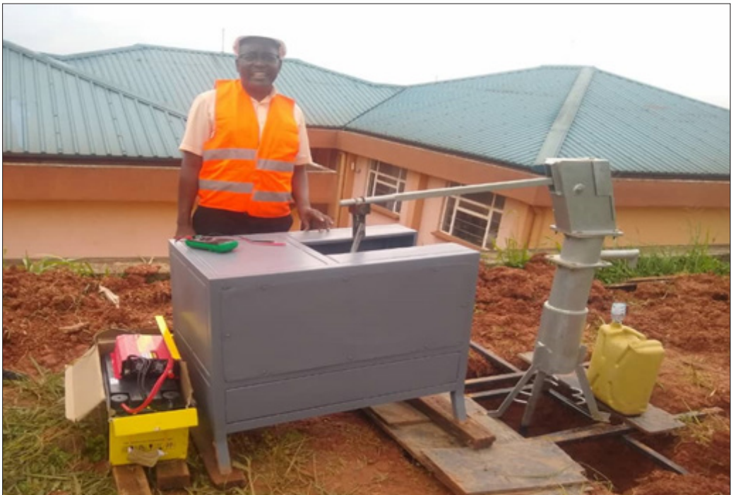
The MAK NAI Borehole
