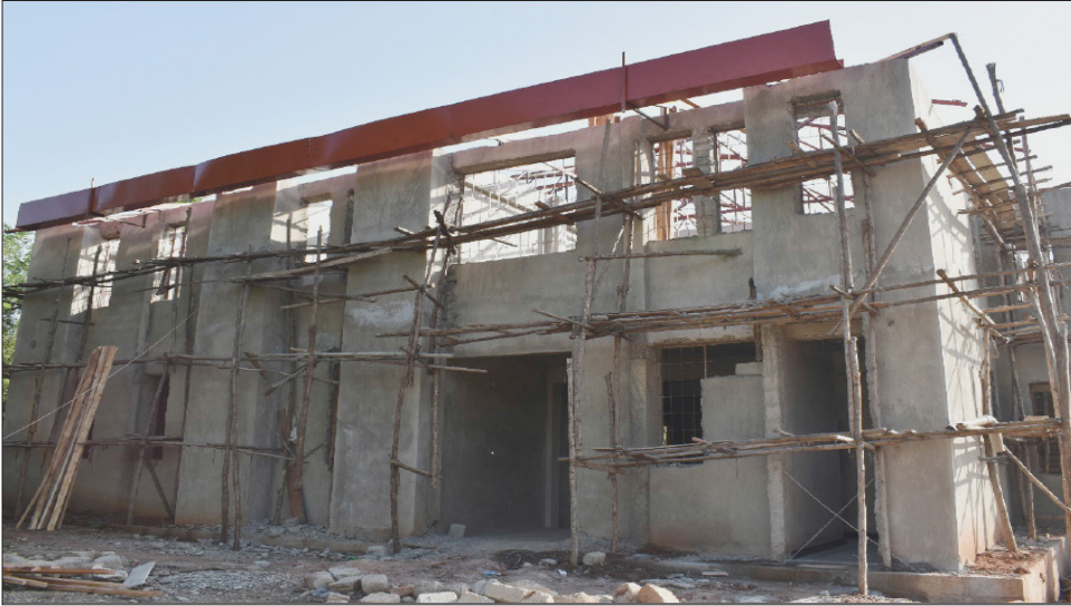
Structure of the MaRCCI building under construction
