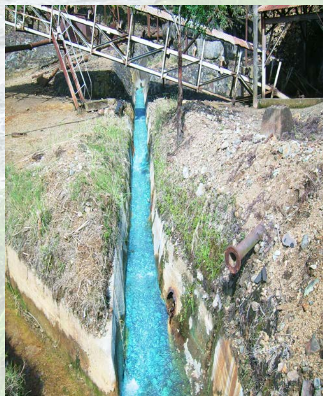
Underground mine water contributes acidity and metals into Kilembe soils and water
