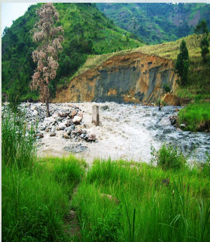
Location of tailings along River Nyamwamba leads to tailing erosion by the river
