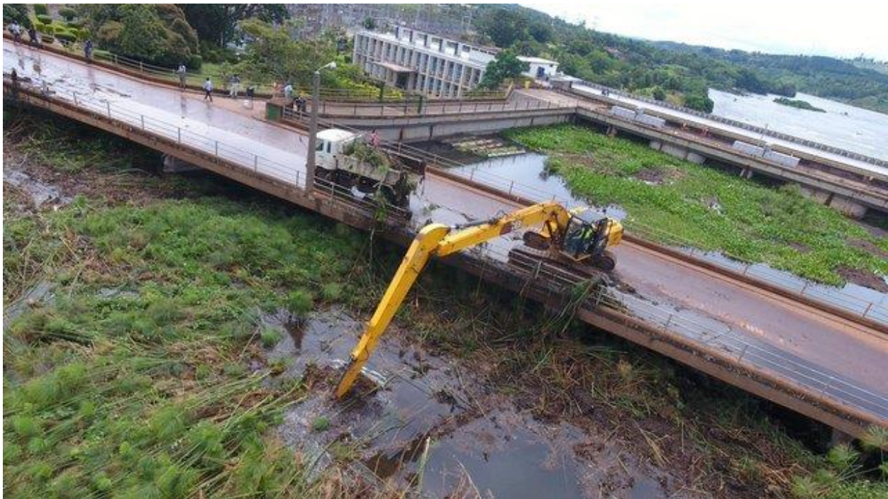
Disintegrated and floating vegetation that choked the Jinja Hydro Electricity Power station early this year
