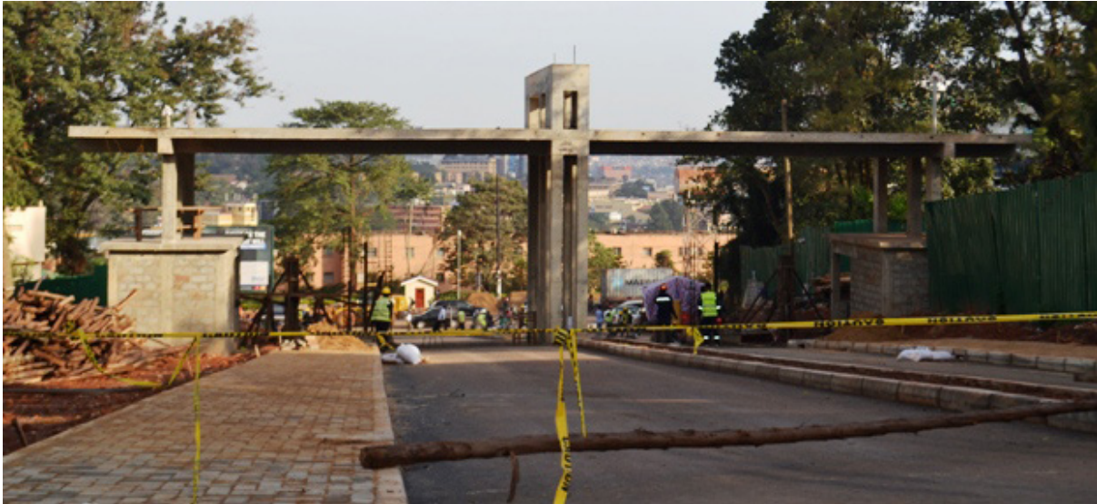
Latest images of ongoing works at the Makerere University Main Gate under the Mak/KCCA MoU
