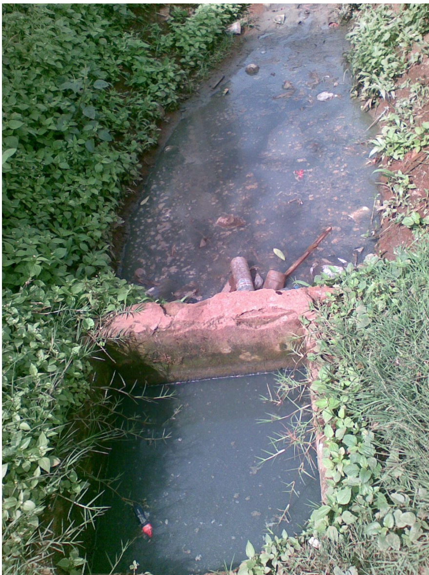
Figure 5: Stagnant kitchen wastewater of a blocked drainage manhole at Mitchell Hall of residence, Makerere University.
