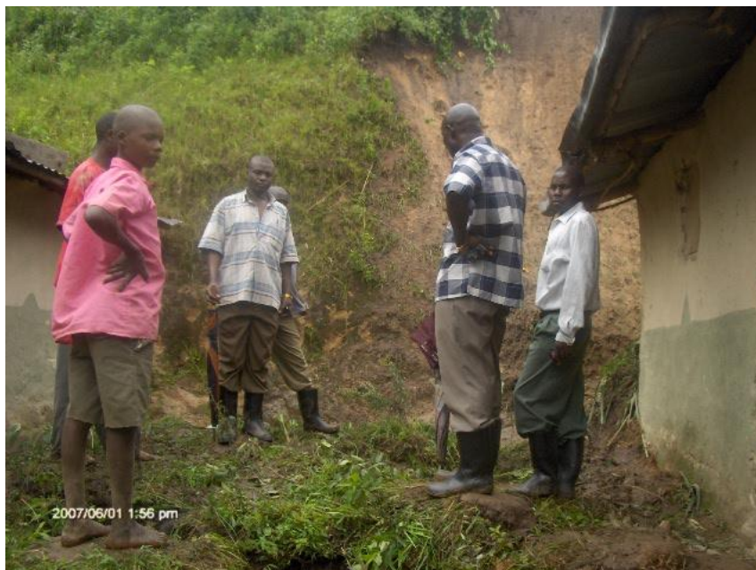
Figure 10: This landslide due to house construction killed two children in 2007.
