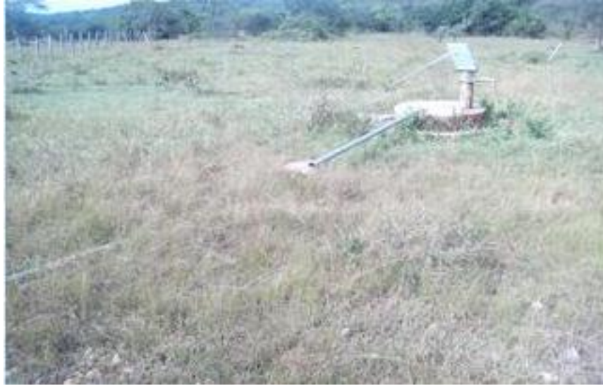
Fig 4.6: Broken hand Pump on Lwanamboga Valley Tank
