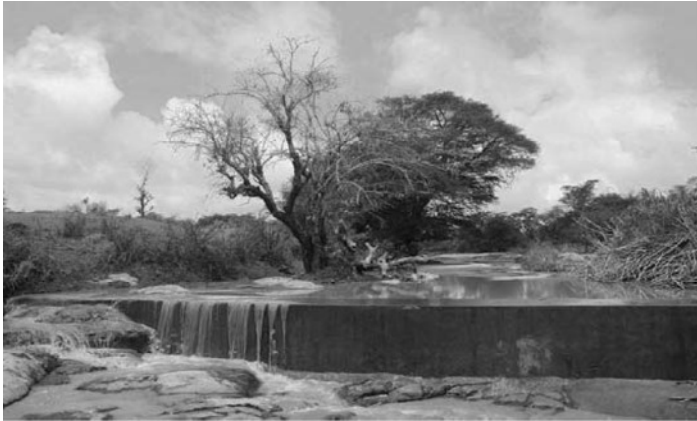
Fig. 1: Sand storage dam in Kitui (Source: Borst and de Hass)
