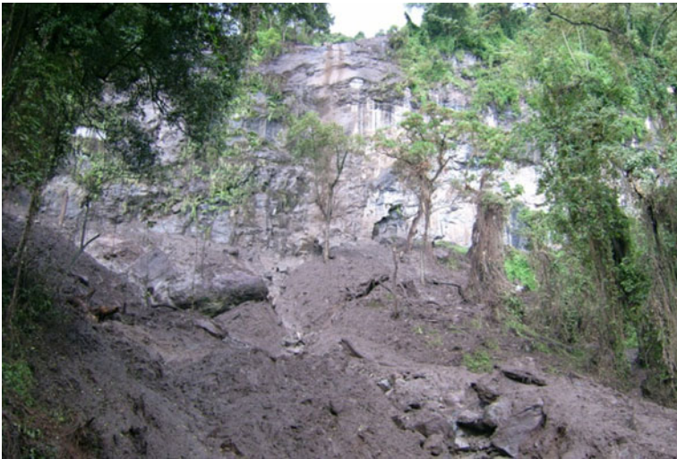
Fig. 3 Part of the Kitati landslide site on the pristine densely forested slopes of Mt. Elgon National Park
