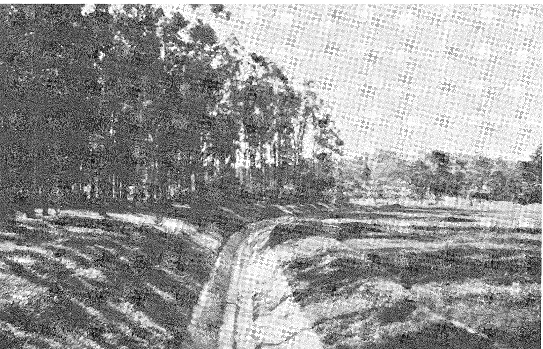
Fig. 8.--A valley that has been drained, with runoff channelized as shown. Trees are planted to absorb water.
